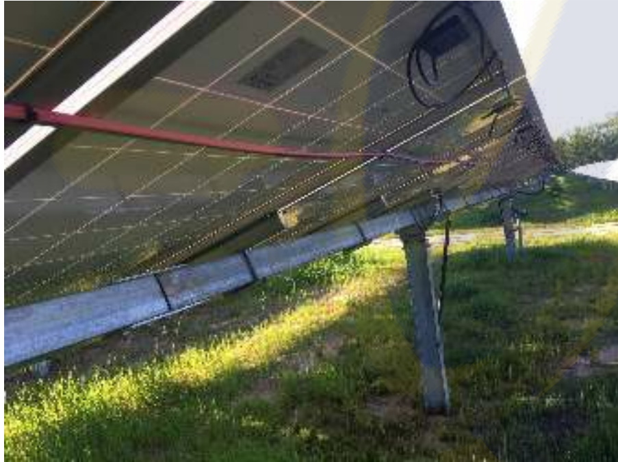
Remove DC wire and open connectors between DC modules.
