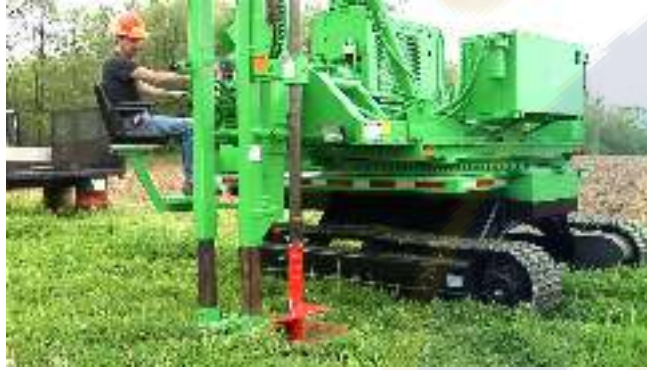
GRT Pile driver
